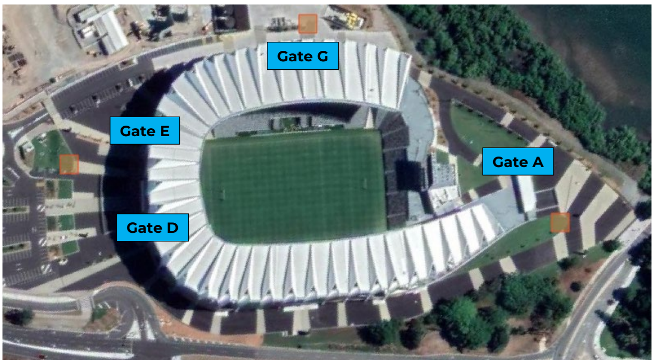
Figure 4 - Red squares indicate the locations of the DOSAs at Queensland Country Bank Stadium
