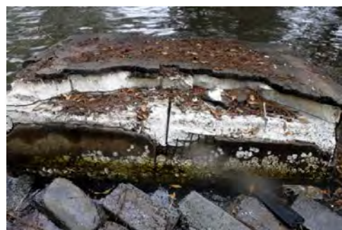
Polystyrene leaking from this pontoon in Cogra Bay
